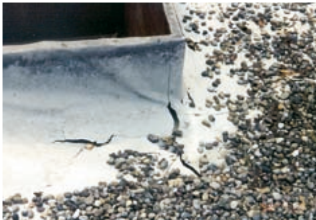
Figure 6.13: Lé d'étanchéité vieilli, photo GVL.
