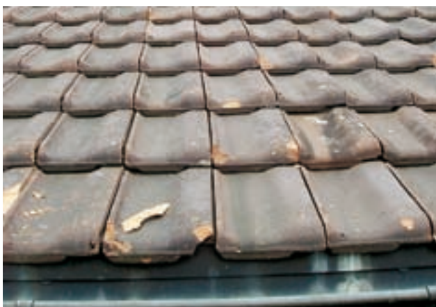
Figure 6.1: Tuiles flamandes, photo GVZ.
